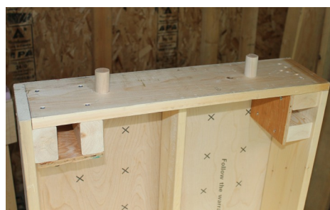
Photo 3- Short pieces of one inch dowel are in place
